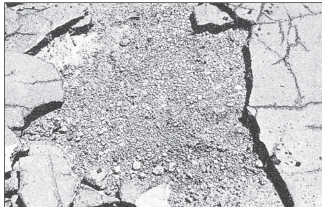
Below - Examples of damage caused by trapped sub-surface water
