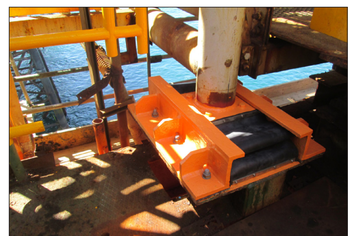
Bearing replaced complete with protective cover
