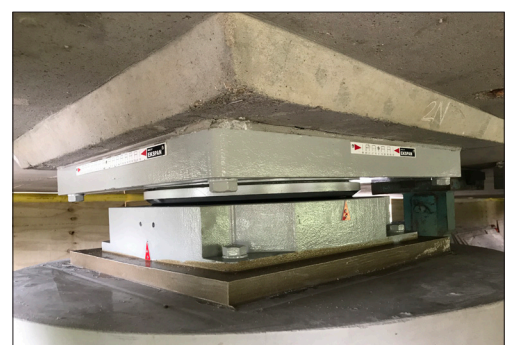
Spherical bearing installed
