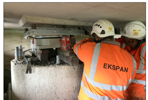
Bonding of top of bearing to the bridge structure
