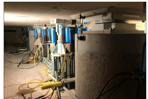
Temporary works and jacking of bridge column during bearing installation
