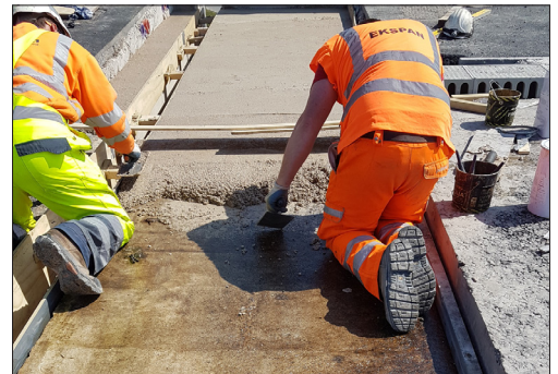
Installing of leveling screed onto concrete bed before lifting the TF joint planks into position
