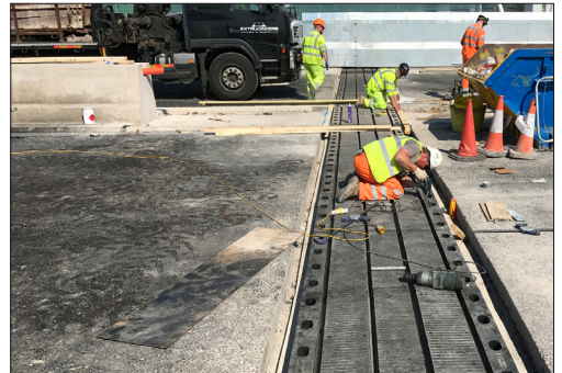
Bolting of TF expansion joint planks along the carriageway
