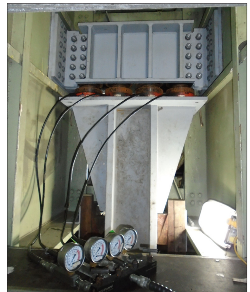
Jacking of twin bridge beams with bespoke temporary works
