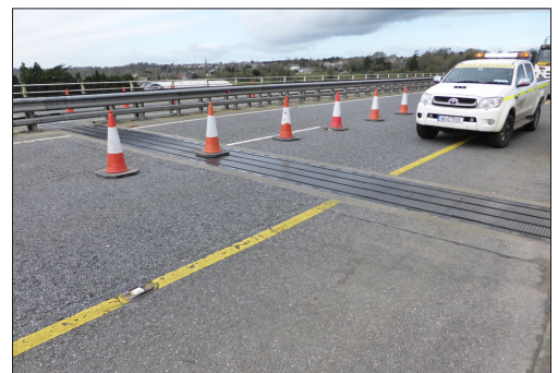
Completion of replaced expansion joint
