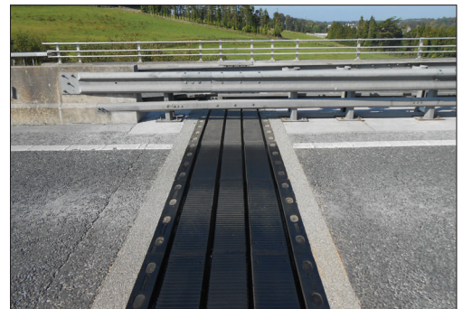
New installed TF1300 expansion joint
