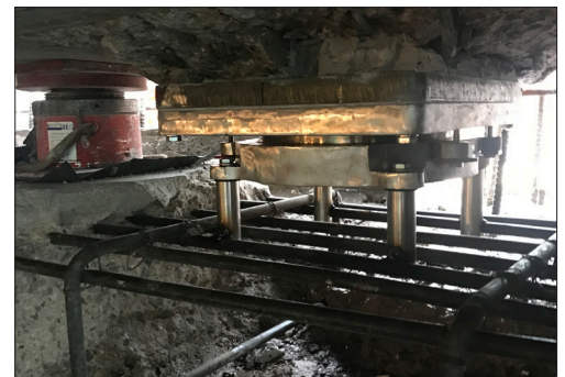
Temporary jacks, hydro demolition and bearing installation
