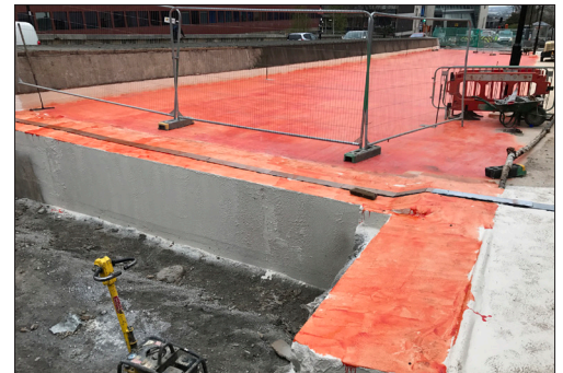
Water proofing applied to the bridge deck
