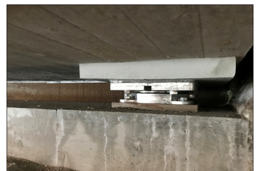
New installed pot bearing
