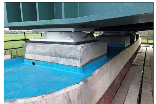
New installed pot bearings on pier top with added concrete protection.
