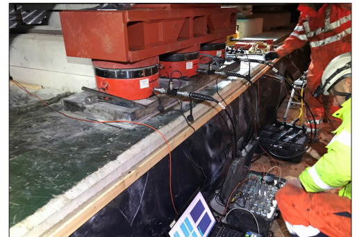
Hydraulic jacking assembly digitally monitors and controls the bridge's movement during bearing removal and replacement.
