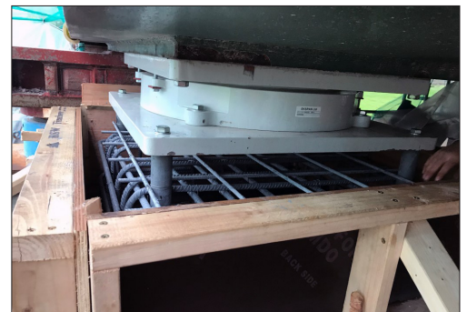
Installation of steel rebar and shuttering in place to accept pouring of concrete for the new bearing plinth.
